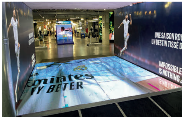
Installation de sol LED Flagship Adidas, Paris (2022)
